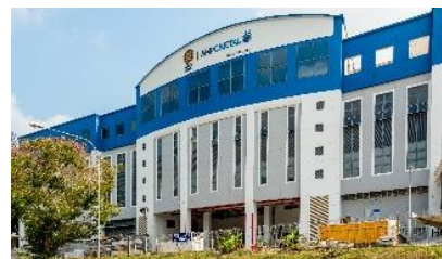
11 Changi South Street 3
