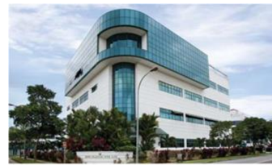
541 Yishun Industrial Park A
