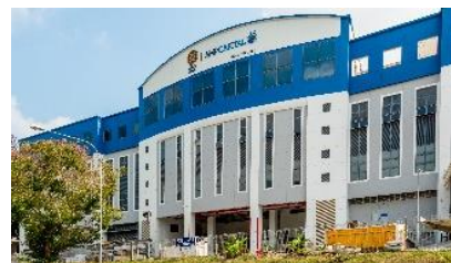
11 Changi South Street 3
