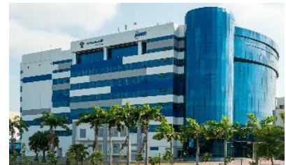
10 Changi South Lane
