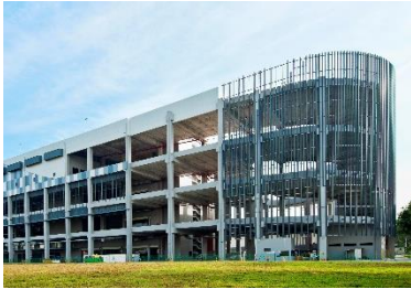
3 Tuas Avenue 2, Singapore
