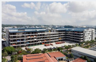
To be installed atop 20 Gul Way, Singapore
