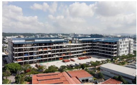
Solar panel to be installed atop 20 Gul Way, Singapore
