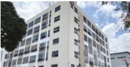
20 61 Yishun Industrial Park A
