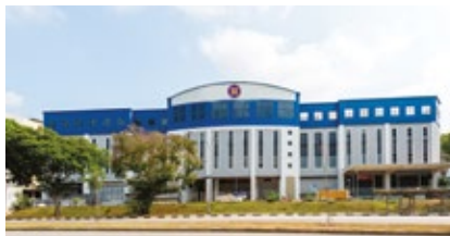
8 11 Changi South Street 3
