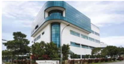
24 541 Yishun Industrial Park A
