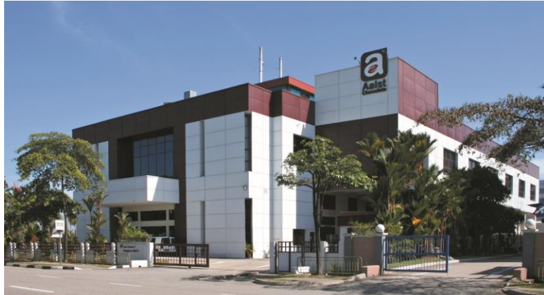
26 Tuas Avenue 7, Singapore
