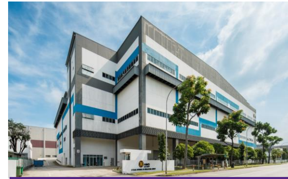
8 Tuas Avenue 20, Singapore
