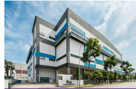
8 Tuas Avenue 20, Singapore
