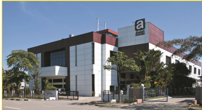
26 Tuas Avenue 7, Singapore
