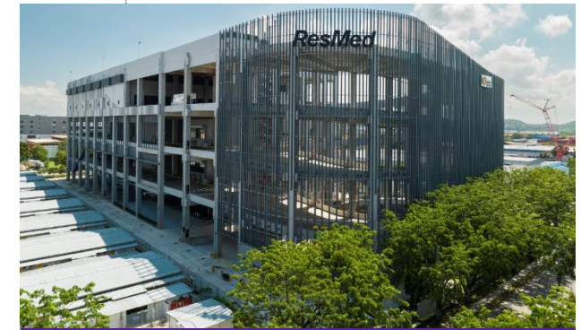
3 Tuas Avenue 2, Singapore
