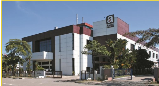
26 Tuas Avenue 7, Singapore
