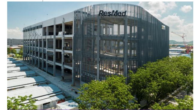
3 Tuas Avenue 2, Singapore
