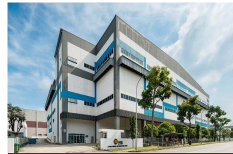
8 Tuas Avenue 20, Singapore
