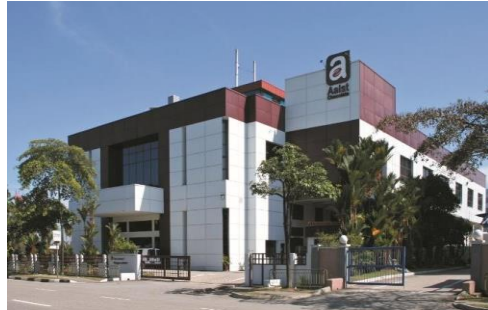
26 Tuas Avenue 7, Singapore
