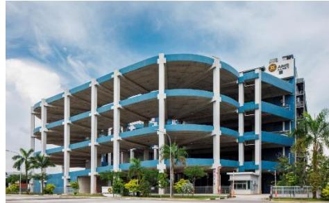
30 Tuas West Road, Singapore
