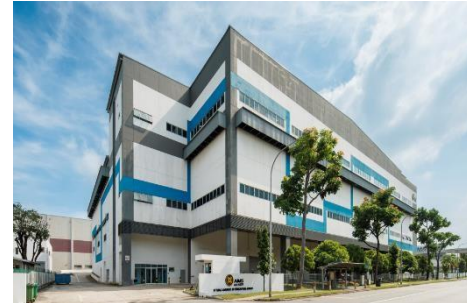
8 Tuas Avenue 20, Singapore
