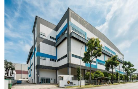
8 Tuas Avenue 20, Singapore
