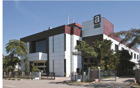
26 Tuas Avenue 7, Singapore
