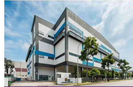
8 Tuas Avenue 20, Singapore
