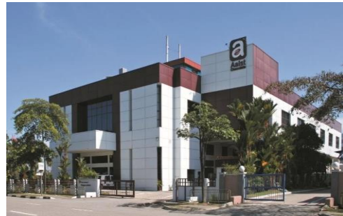
26 Tuas Avenue 7, Singapore
