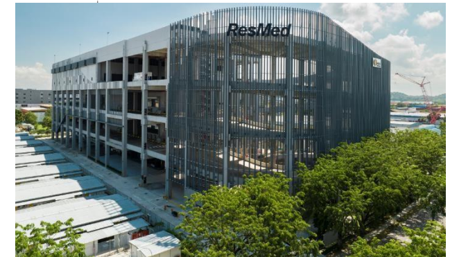
3 Tuas Avenue 2, Singapore
