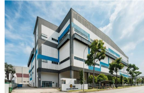
8 Tuas Avenue 20, Singapore
