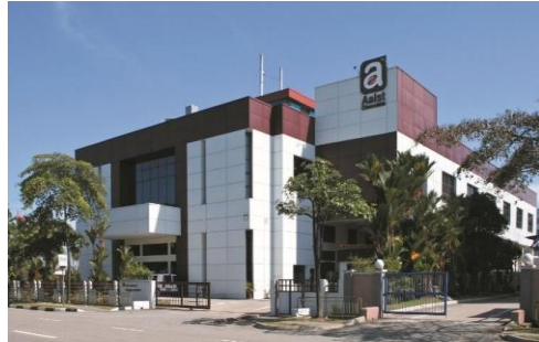
26 Tuas Avenue 7, Singapore
