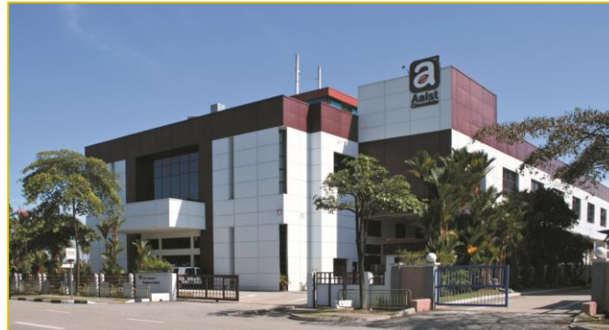
26 Tuas Avenue 7, Singapore
