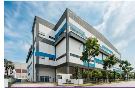
8 Tuas Avenue 20, Singapore
